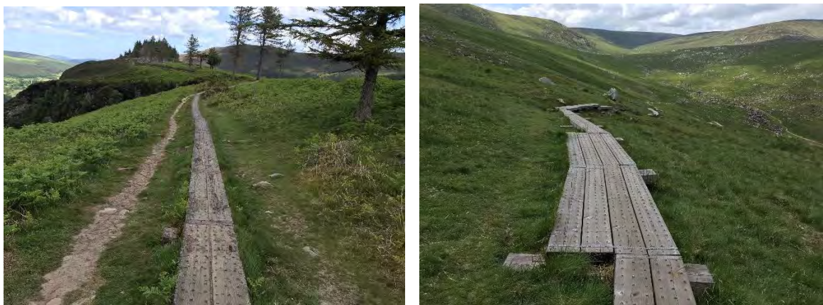
Fig. 21 Damaged surface running parallel to the boardwalk where it's not wide enough for walkers to pass. Where the boardwalk has been widened this is having a positive impact.
