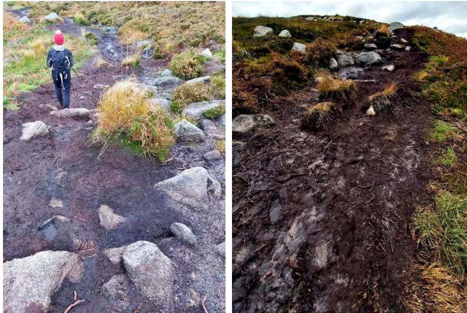
Fig. 31 Erosion damage on the steeper slopes of the glacial moraine. Surface of path devoid of vegetation cover exposing peaty soils much of which is being washed away by natural erosion processes leaving a slippery, wet path for walkers to navigate and causing increased path erosion.
