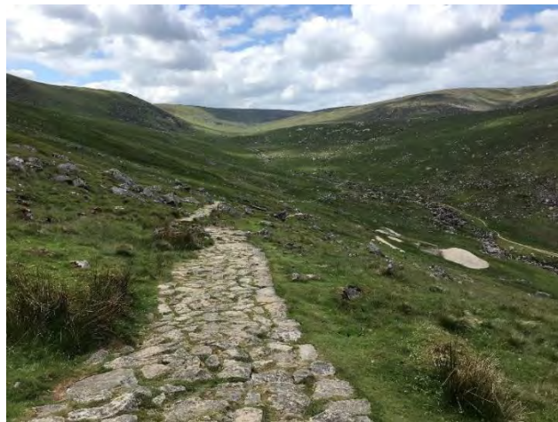
Fig. 19: Previously eroded trail that has been stone paved just after where the boardwalk stops
